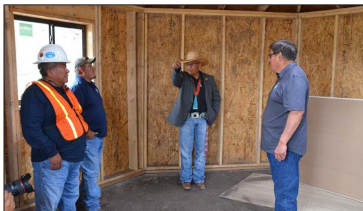
PHOTO: Speaker LoRenzo Bates and Council Delegate Steven Begay visit a hogan under construction in Naschitti, N.M. on Aug. 21, 2018.
