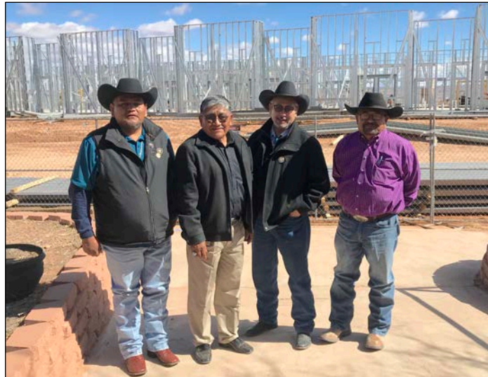
PHOTO: (left to right) Council Delegates Davis Filfred, Leonard H. Pete, Benjamin L. Bennett, and Lee Jack, Sr. at the construction site of the new Chinle Nursing Home facility in Chinle, Ariz. on Feb. 28, 2018.
