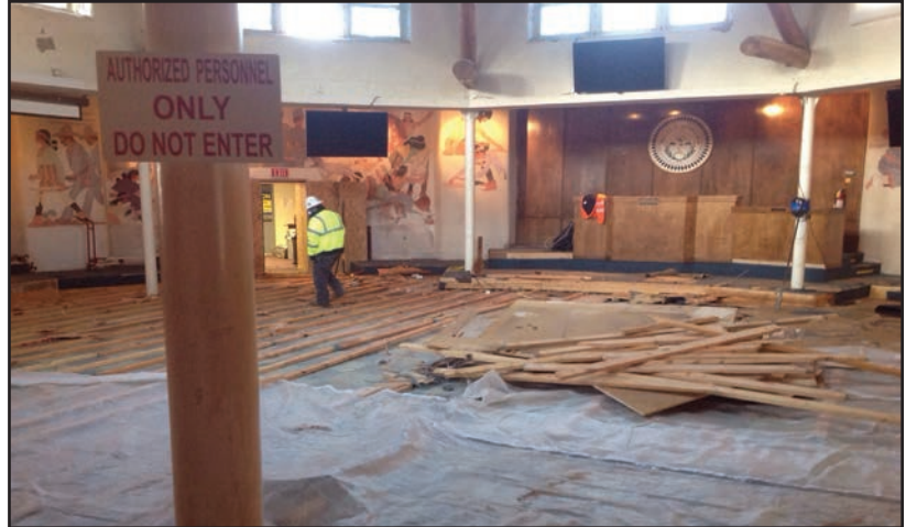
Photo: Demolition of Navajo Nation Council Chamber floor. (Dec. 8, 2016)
