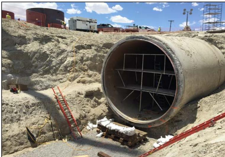
**PHOTO: Contractors continue to make progress on the replacement of the 40-foot portion of the pipe on May 30, 2016 (Photo courtesy of the Bureau of Reclamation).**
