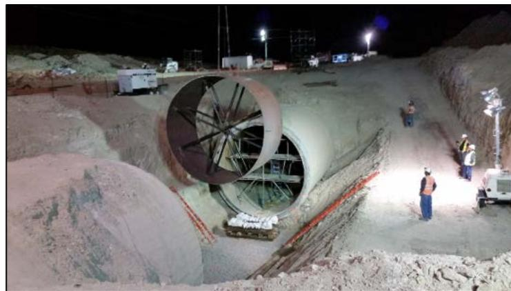
**Photo: The first section of pipe being lowered into place at the breach site on May 29, 2016 (Photo courtesy of the Bureau of Reclamation).**
